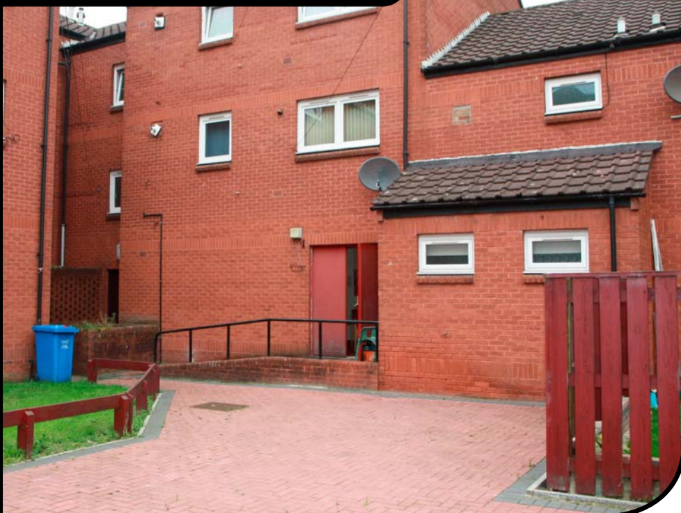
REAR EXTERIOR BEFORE
