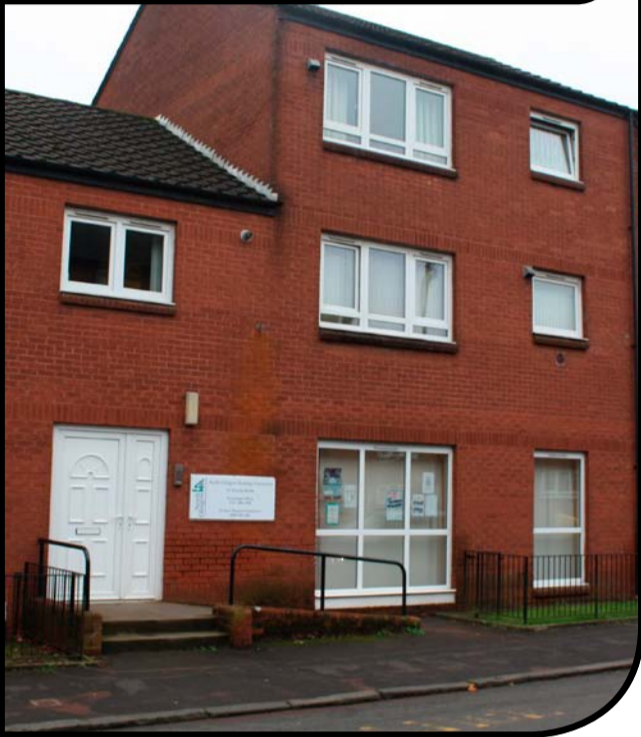
FRONT EXTERIOR BEFORE
